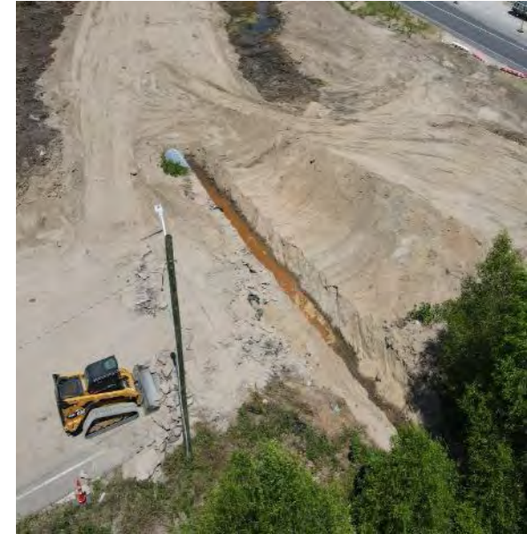
Drainage Pipe Relocation
